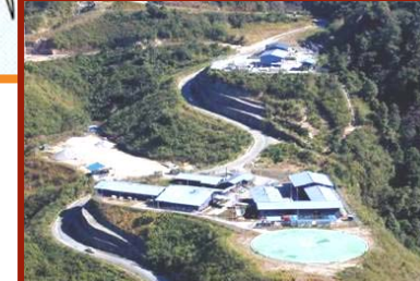
Metering Station (MS)
